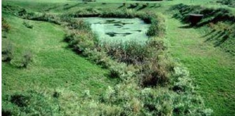
Figure 2. An example of an extended dry detention pond – Modified from http://www.vwrrc.vt.edu/swc/NonPBMPSpecsMarch11/VASWMBMPSpec15EDPOND.html .
